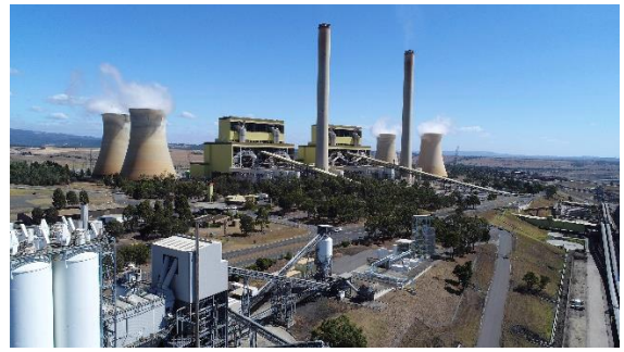
Brown coal hydrogen production plant, © HySTRA
